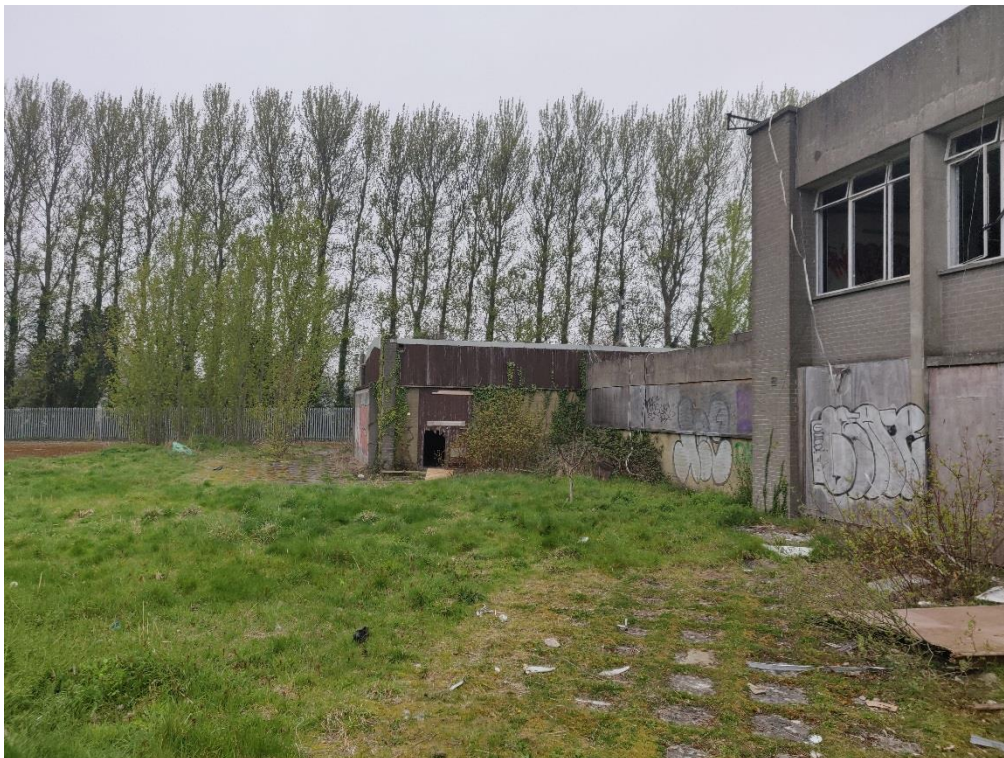
Figure 6.5 – End of Building 3 & 4: Storage Warehouse: East Elevation
