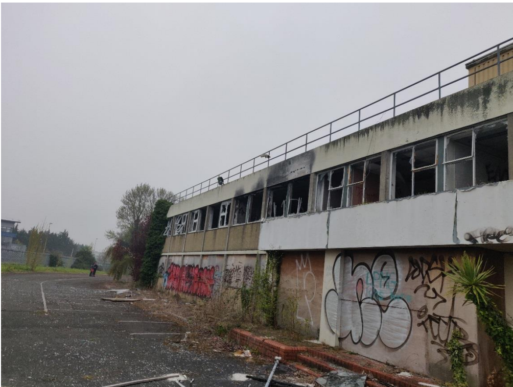
Figure 6.3 – Building 2: East Elevation
