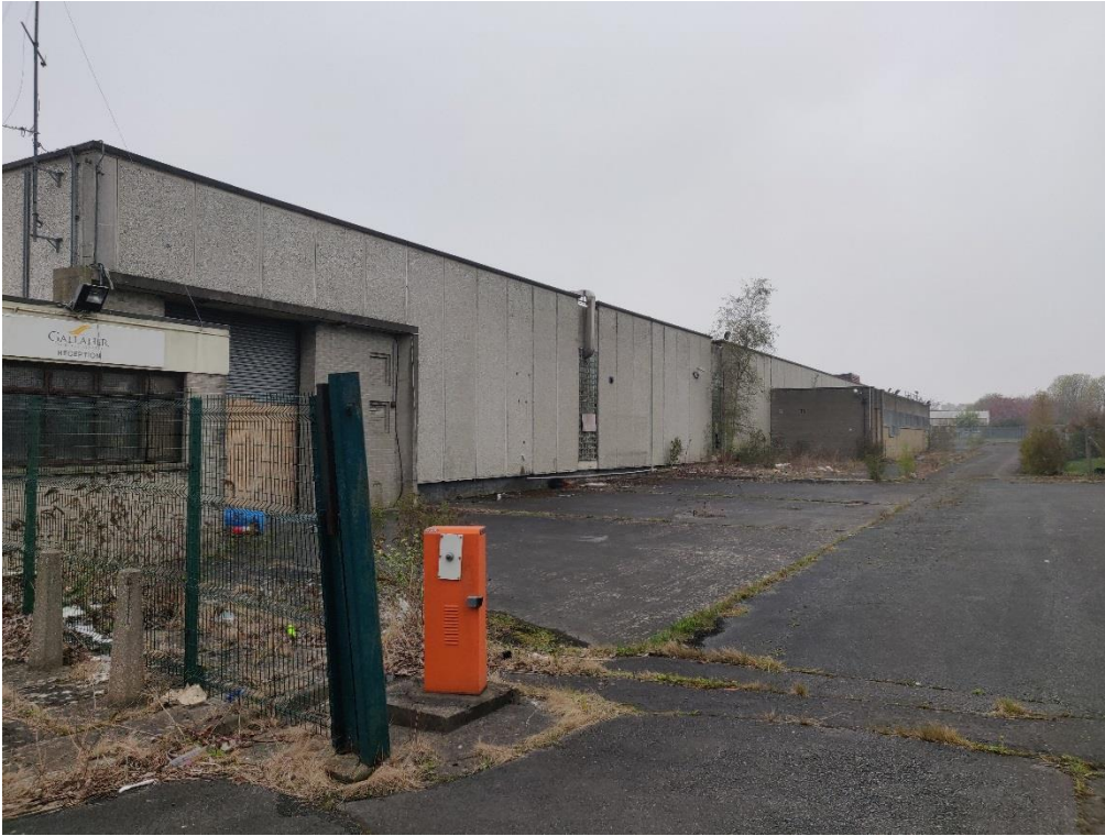
Figure 6.2 – Building 1: Factory Warehouse: North Elevation.
